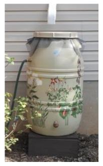
Figure 8a: Rain barrel used to disconnect a downspout with the overflow going to flower bed
