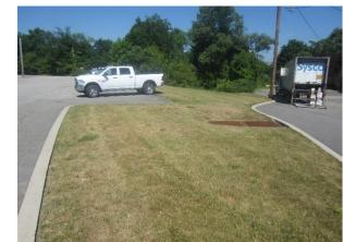
Stormwater is currently directed to an existing catch basin in the grassy medium along the northern parking spaces. A rain garden installed in this grass area can capture, treat, and infiltrate runoff from the lot. A preliminary soil assessment suggests that the soils have suitable drainage characteristics for green infrastructure.
