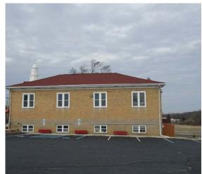
A small rain garden can be installed to capture, treat, and infiltrate runoff from the church's rooftop. A portion of the parking lot runoff can be captured by replacing some parking spaces with pervious pavement. A preliminary soil assessment suggests that the soils have suitable drainage characteristics for green infrastructure.
