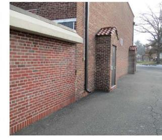
The paved area adjacent to the building can be depaved and replaced with a rain garden to capture, treat, and infiltrate rooftop runoff. Rainwater can be harvested by installing cisterns around the building. The water can then be used for watering gardens, washing vehicles, or for other non-potable uses. A preliminary soil assessment suggests that the soils have suitable drainage characteristics for green infrastructure.
