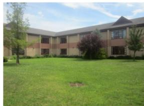
Stormwater is currently directed to existing catch basins. Parking spots by the north and west buildings can be replaced with porous asphalt to capture and infiltrate stormwater runoff from the parking lot. Rain gardens adjacent to the building can capture, treat, and infiltrate roof runoff before it reaches the existing catch basin. A preliminary soil assessment suggests that the soils have suitable drainage characteristics for green infrastructure.
