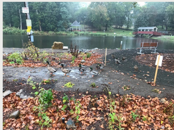
Site after the rain garden installation
