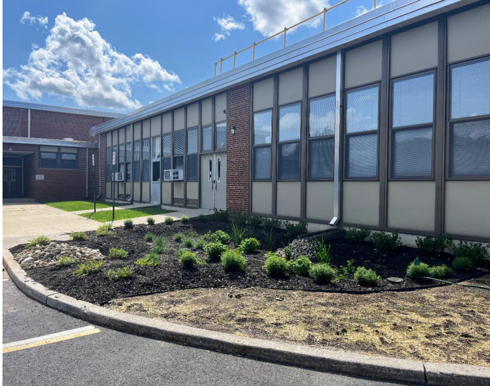
Completed rain garden at Hackettstown High School [Photo credit: Carl Johnson, Hackettstown Board of Education]
