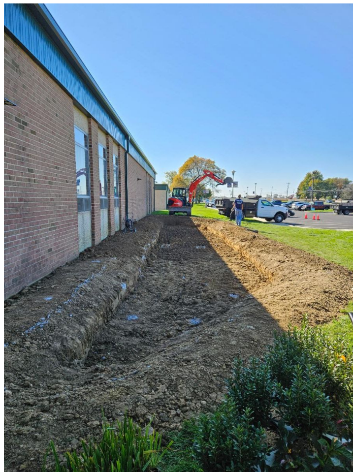
Rain garden construction, November 2023
