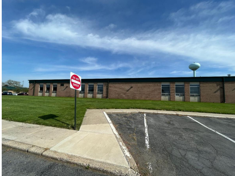
Project site, Salem County Career and Technical High School, Pilesgrove Township
