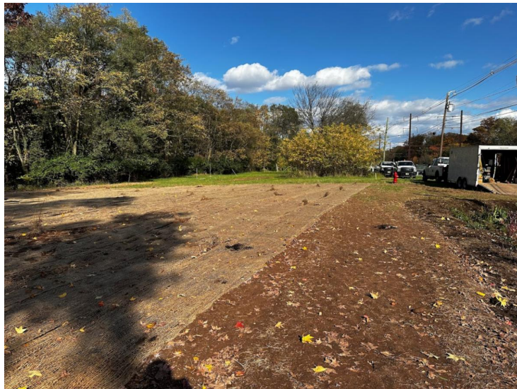
Upland pollinator garden under construction, Woodbridge Township, October 2023
