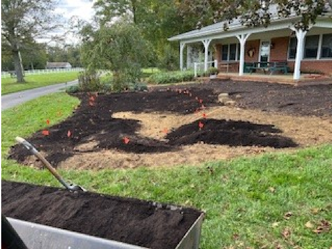
Installation of the rain garden designed as part of the Spring 2023 Homeowner Rain Garden Rebate Program [Photo credit: Roseann Greenberg]
