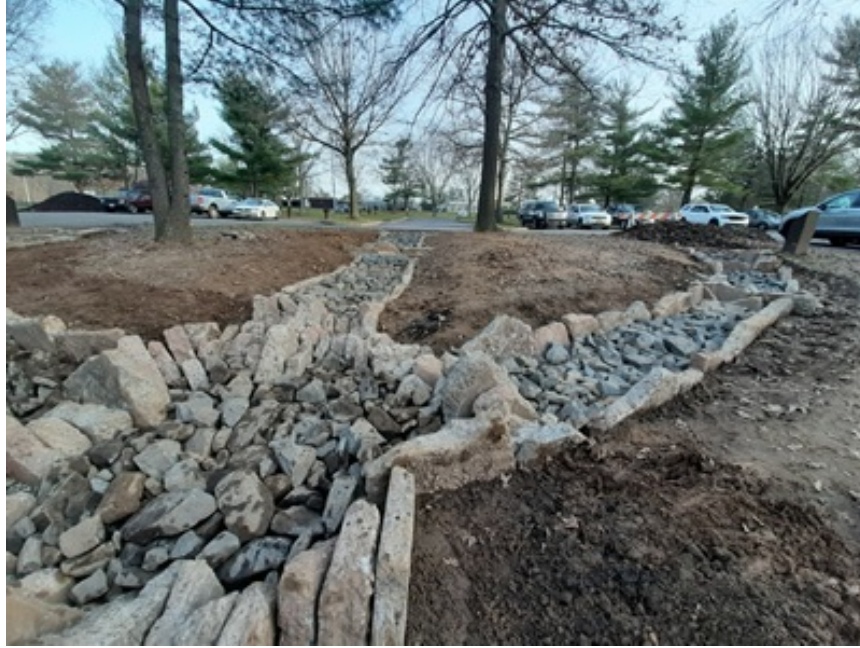
Basin #158 outfall retrofit; December 2020
