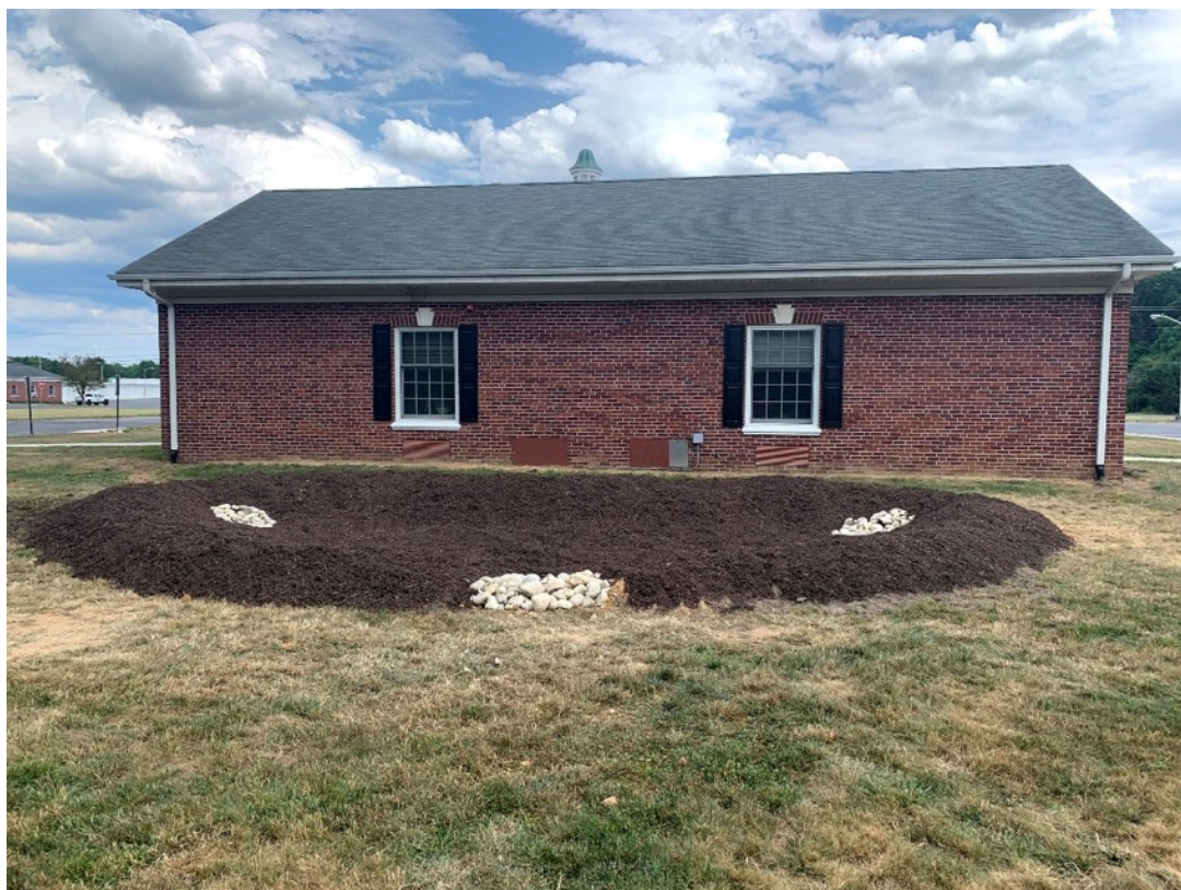
Rain garden construction complete and ready for planting, June 25, 2020
