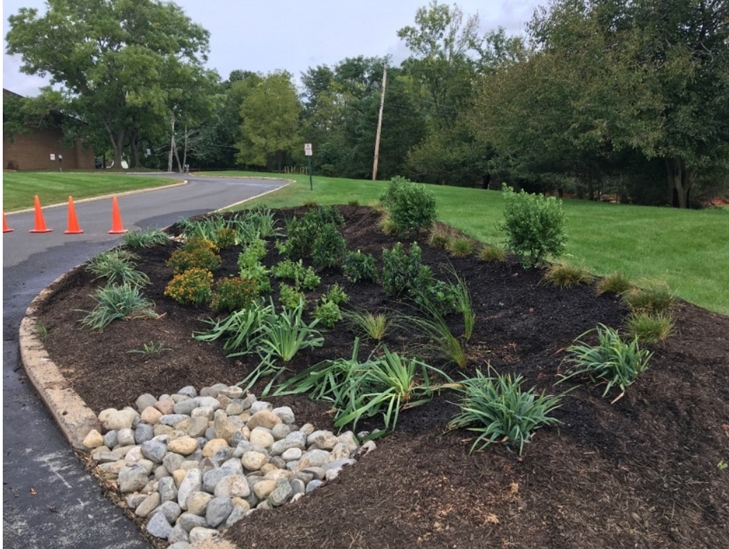
Bridgewater YMCA rain garden following planting, September 2020
