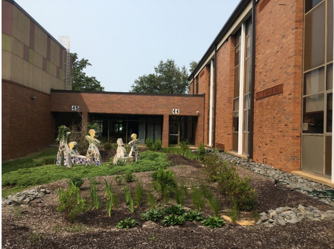
Monroe Township Middle School rain garden, September 16, 2020
