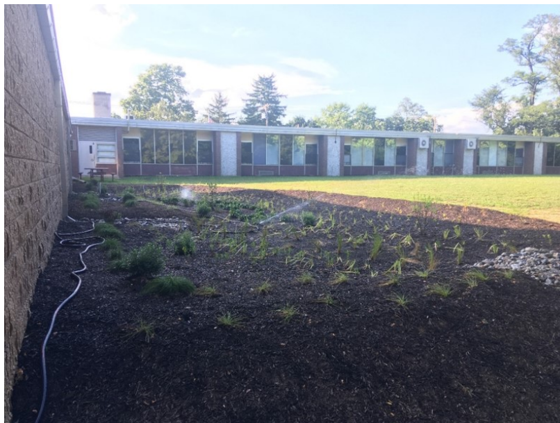
Automatic sprinkler in use at Grace Breckwedel Middle School following the installation of plants, August 1, 2020
