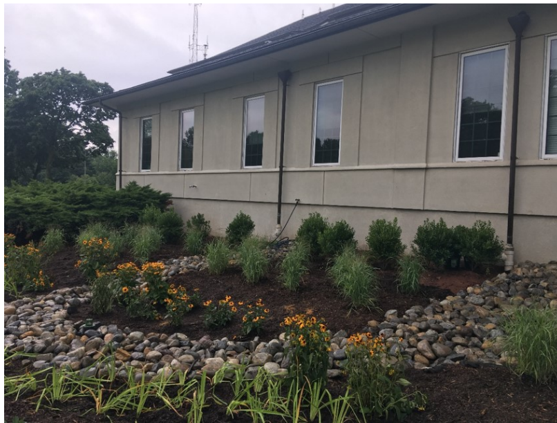
Warren Township Library rain garden, July 2020
