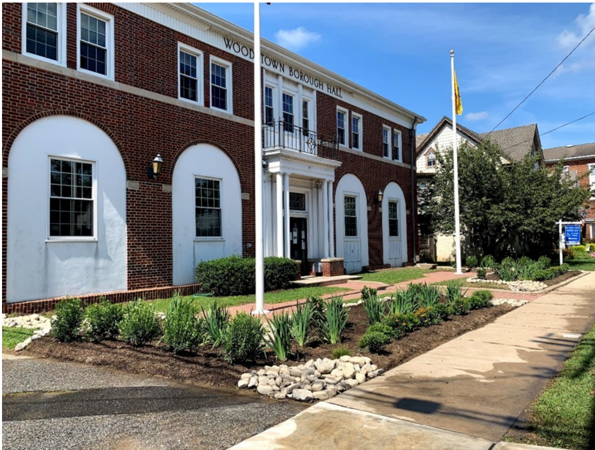
Woodstown Borough Hall rain gardens shortly after planting, August 2020
