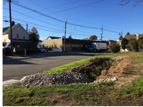
Completed Fulton Street rain garden #4, Woodbridge, NJ
