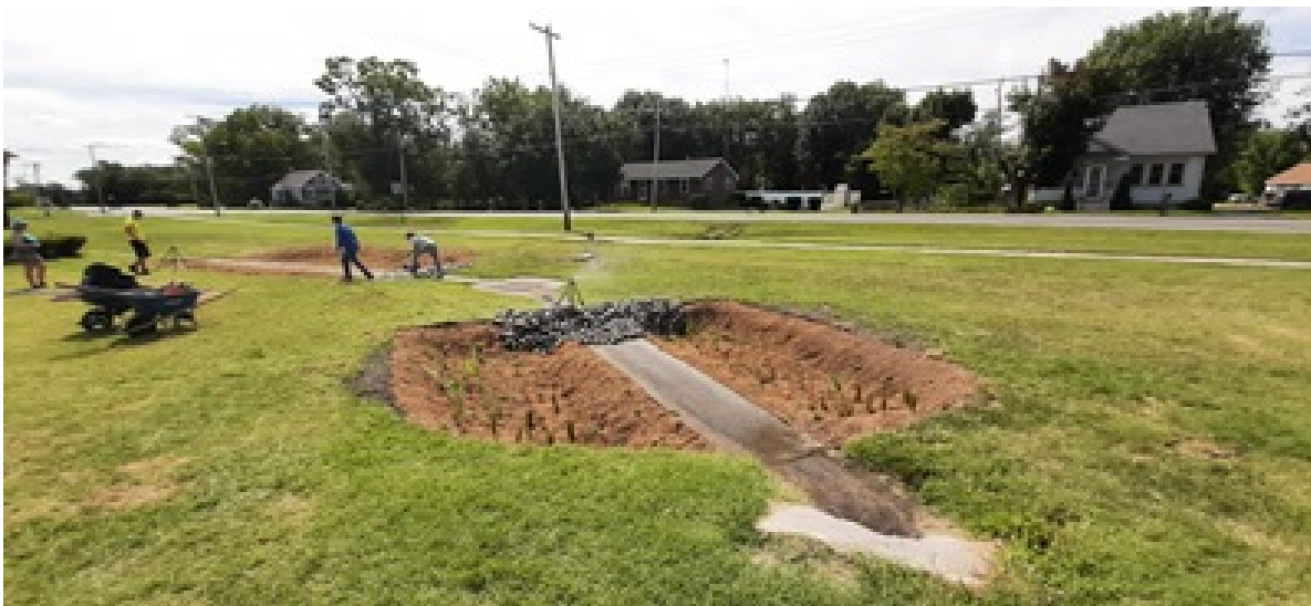
Phase 1: Rain garden installation in the detention basin at Pittsgrove Township Middle School, August 2021
