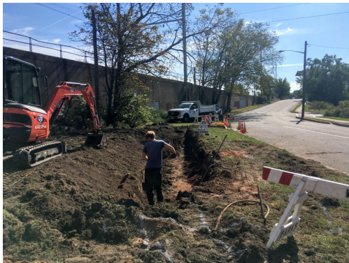
Fulton Street rain garden #4 construction, Woodbridge, NJ
