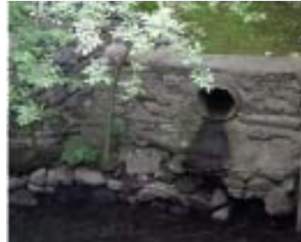
Stormwater outfall pipe.
