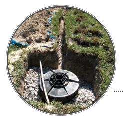
**LOCATION:** Holmdel, NJ. This residential dry well was installed in Monmouth County. It is a underground system that uses an empty container to store large quantities of stormwater during rainfall events.
